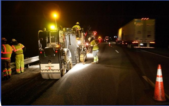
Mill and Overlay
