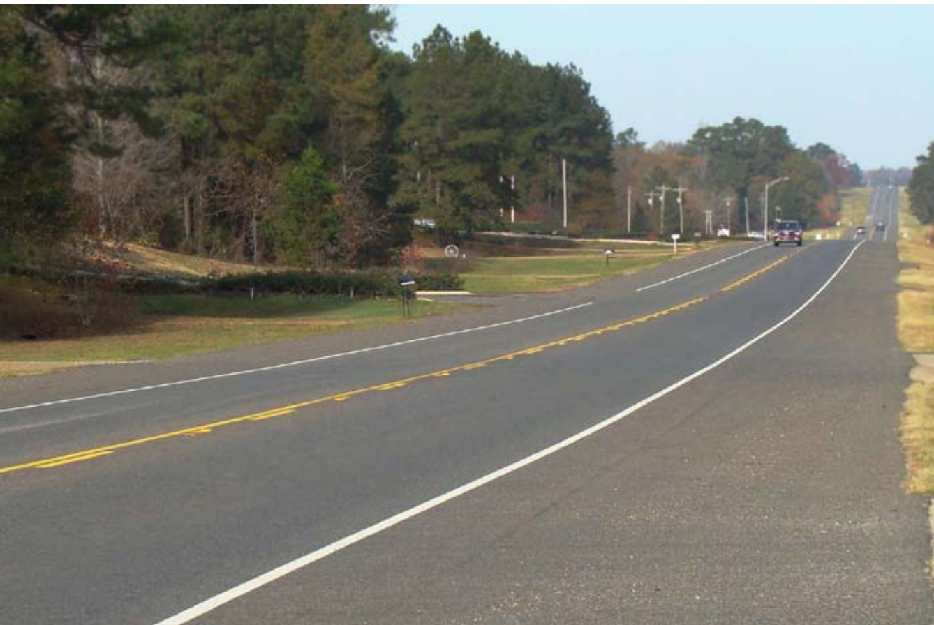
The Kentucky Transportation Cabinet received a 2009 Perpetual Pavement Award for Louisville-Tennessee Road, I-65, Hart County.
