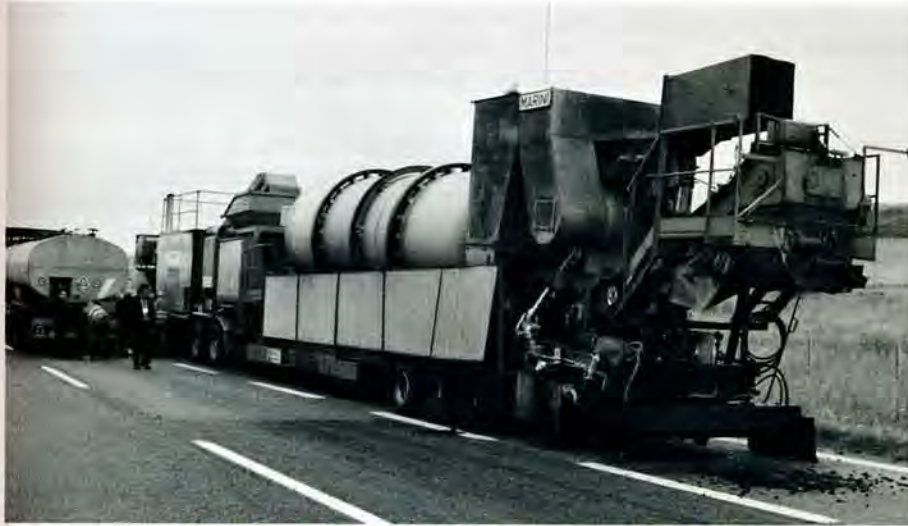
Figure 11. Recycling a porous pavement in Italy.
