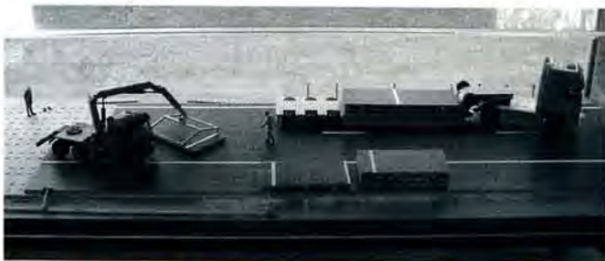
Figure 10. Construction of the ModieSlab (two-layer porous concrete).
