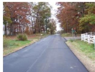
has provided a smooth surface with good friction characteristics. The fine material used in the mix gives an esthetically pleasing look. Current work being performed at the FHWA research facility is documenting the benefits of SM-4.75 in delaying crack initiation.
