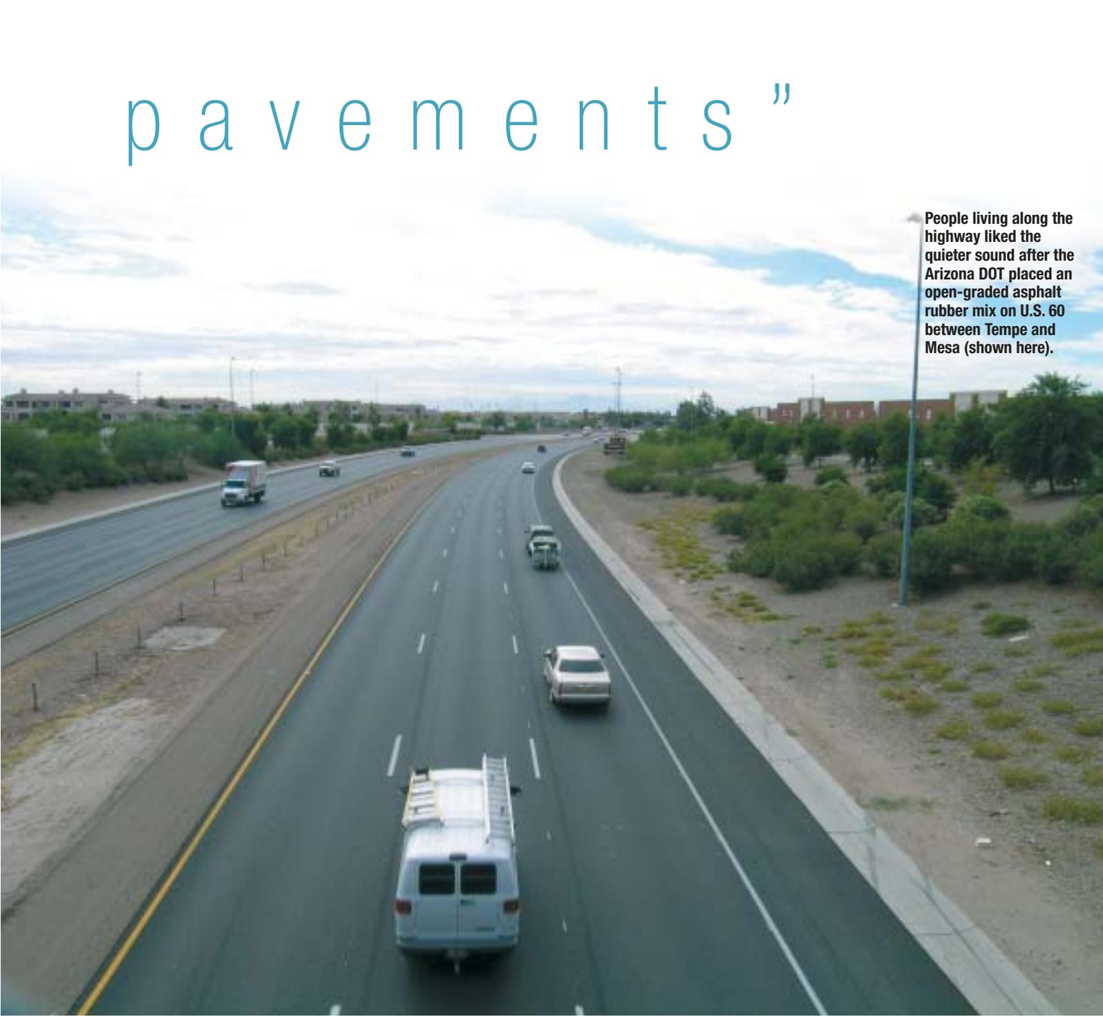
People living along the highway liked the quieter sound after the Arizona DOT placed an open-graded asphalt rubber mix on U.S. 60 between Tempe and Mesa (shown here).
