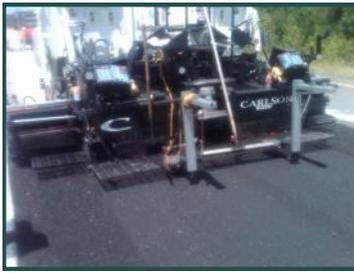
placement of a 5.5" cold recycled base layer. Section 1 was overlaid with 2 inches of IM-19.0D and 2 inches of SMA. For Sections 2 and 3, the cold recycled base layer was laid on a compacted aggregate sub-base. The base layer was a uniform 5.5 inches. Section 2 was overlaid with 4 inches of IM-19.0D and 2 inches of SMA. Section 3 was overlaid with 2 inches of IM-
