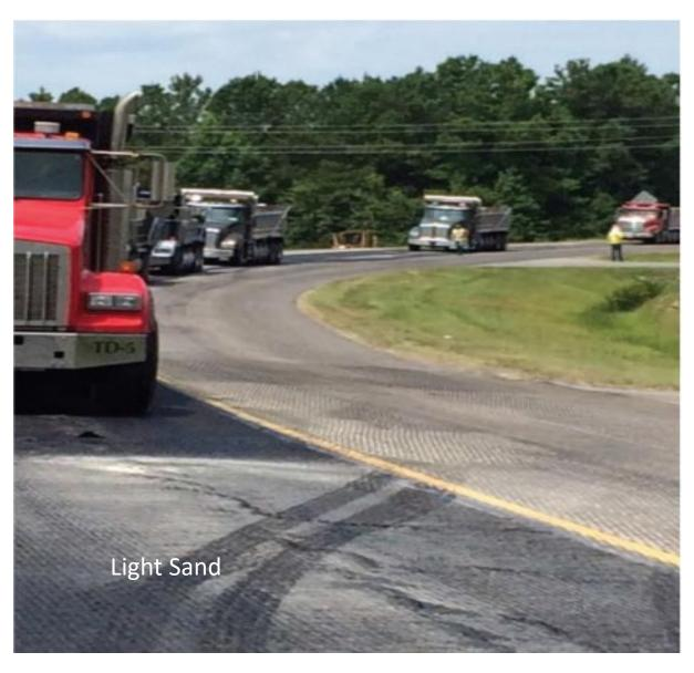
Reinforcement should be durable allowing construction equipment to line up to the asphalt paving machine without "pick-up" under construction truck tires... or paver ...minimizing field construction issues.
