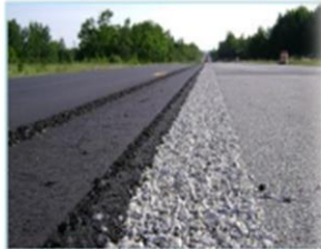
FiberMat® visible at center joint was exposed to 4th of July holiday weekend traffic with no reported issues
